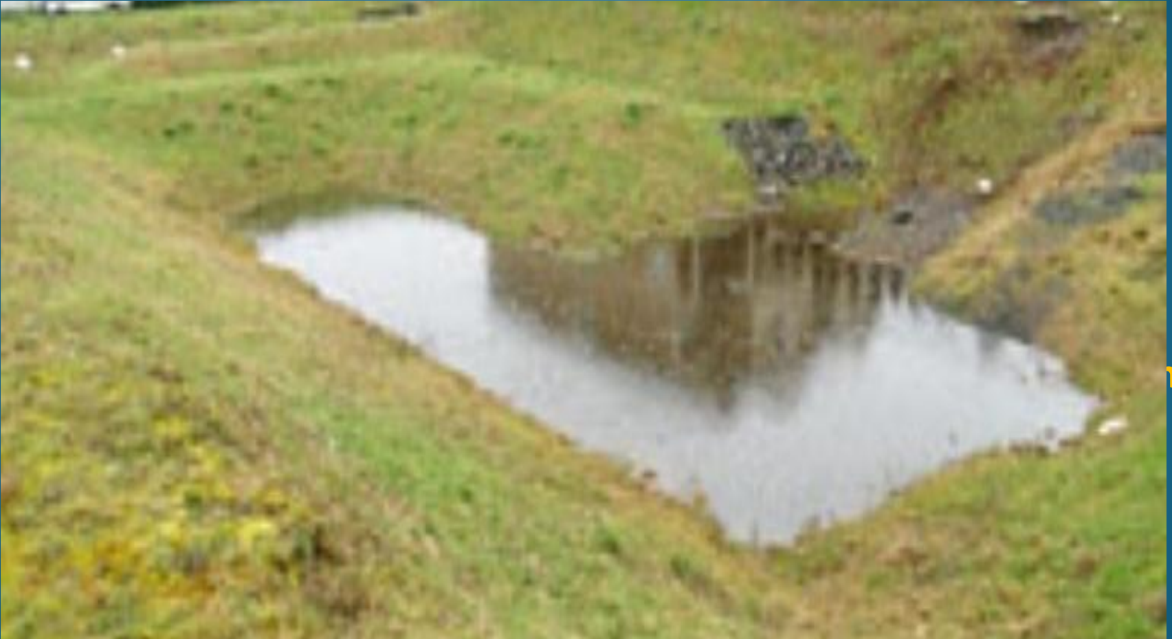
A typical infiltration basin
